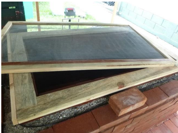
Screen cover to prevent rodents in Guatemala City, Guatemala
