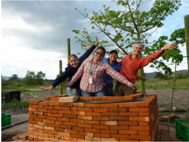
A completed ZECC in Honduras, with cover, water bag and thatched shade structure. A shade curtain was later attached to the sunny side.
