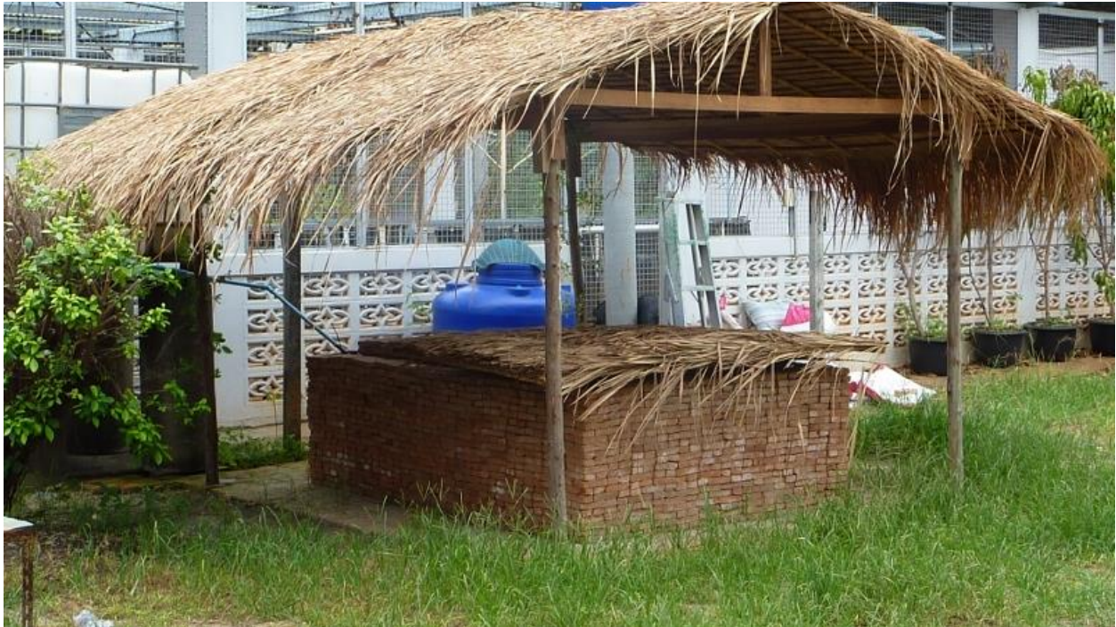
The tiny size of the bricks available in Bangkok, Thailand made ZECC construction costly and time consuming (over 5000 bricks were used: brick size: 13.5cm x 6.0 cm x 3.0 cm)
