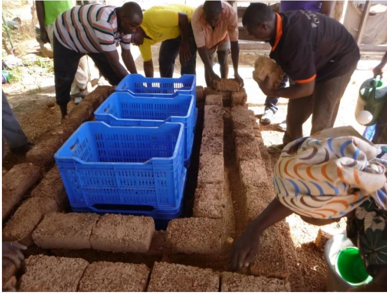
ZECC construction in Ghana
