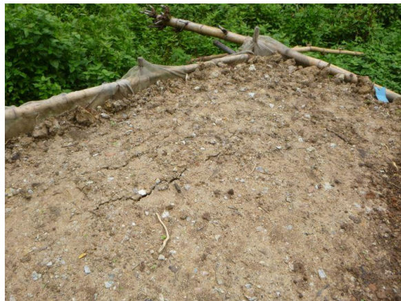
Sloped site being filled and leveled in Chiang Mai in June, but already slumping and cracking in July, causing ZECC to lean and have shorter lifespan.
