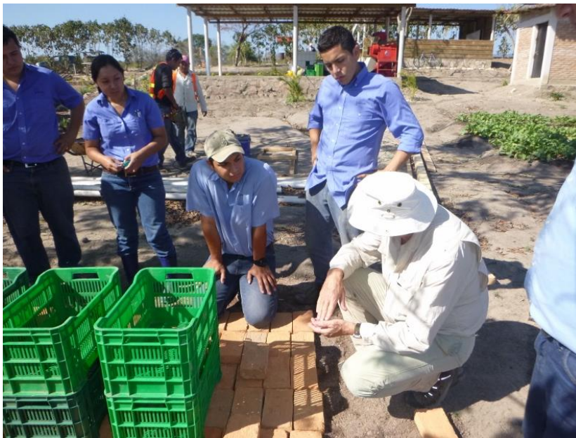
ZECC construction in Honduras
