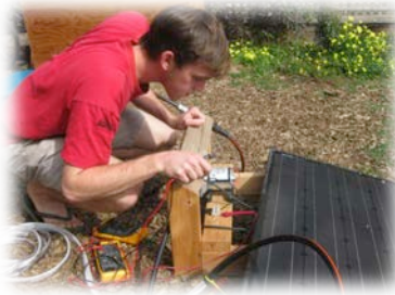
D-Lab student assesses solar panels
